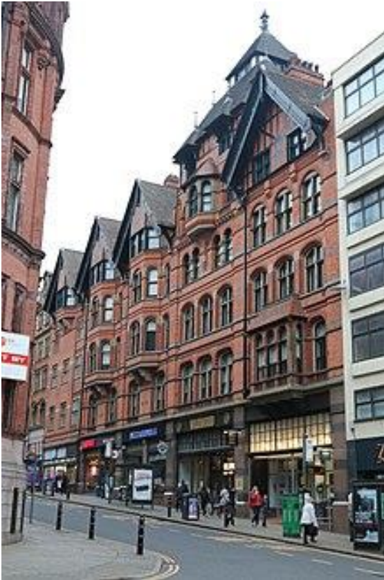
Jessops' Shop and Workrooms, 14–30 King Street, Nottingham – 1894–1897
